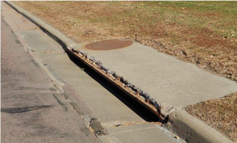
(Photo is a storm inlet in need of repairs on Southeastern Avenue.)
