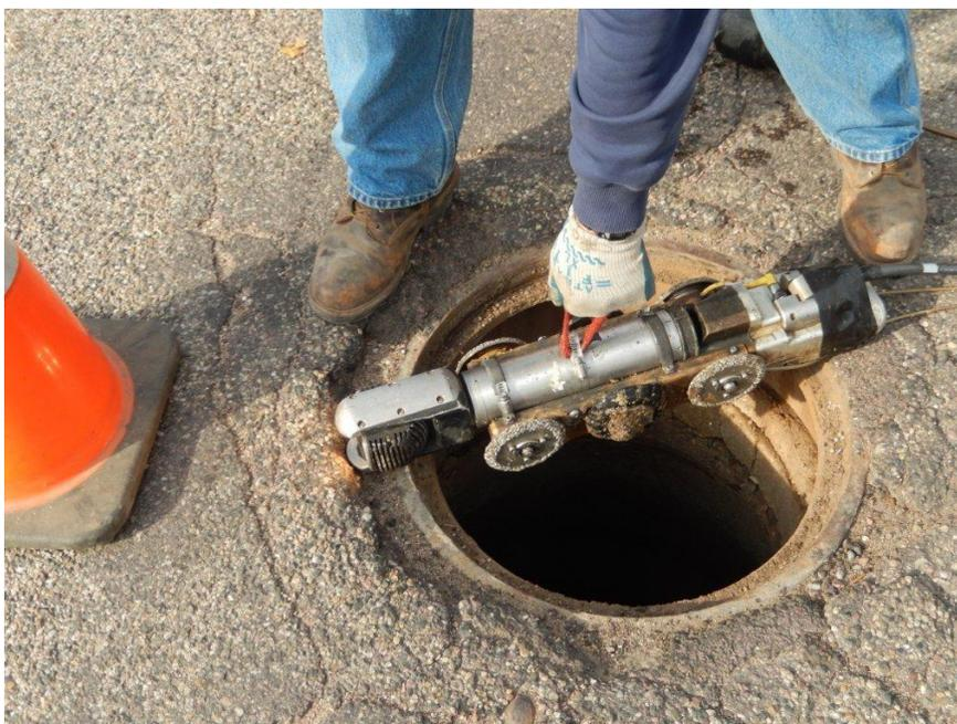
(Photo is that of a City employee preparing to lower a closed circuit video camera into a stormwater line for visual inspection of the condition of the line. Approximately 20% of the lines are video recorded each year with a goal of inspecting the entire system every 5 years.)
